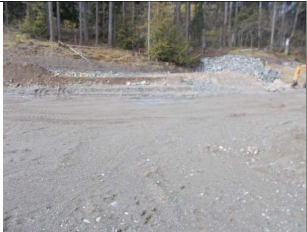
Apr. 1, 2023: Current condition of Lot 50, with pit run sand and gravel exposed as subgrade.
