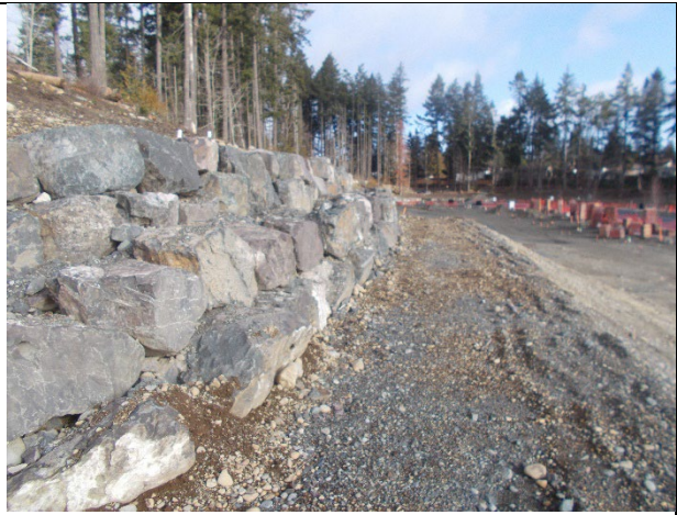
Mar. 15, 2023: Tiered boulder wall constructed at rear of Lot 40, to be left in place.
