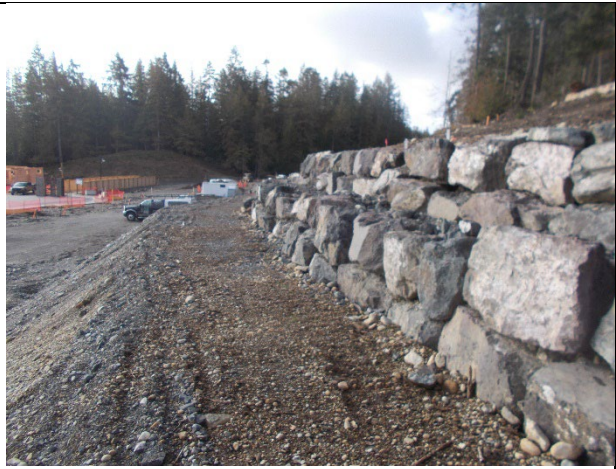
Mar. 15, 2023: Tiered boulder wall constructed at rear of Lot 42, to be left in place.
