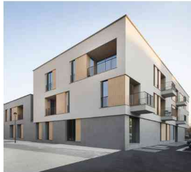
SMOOTH STUCCO APPLICATION
