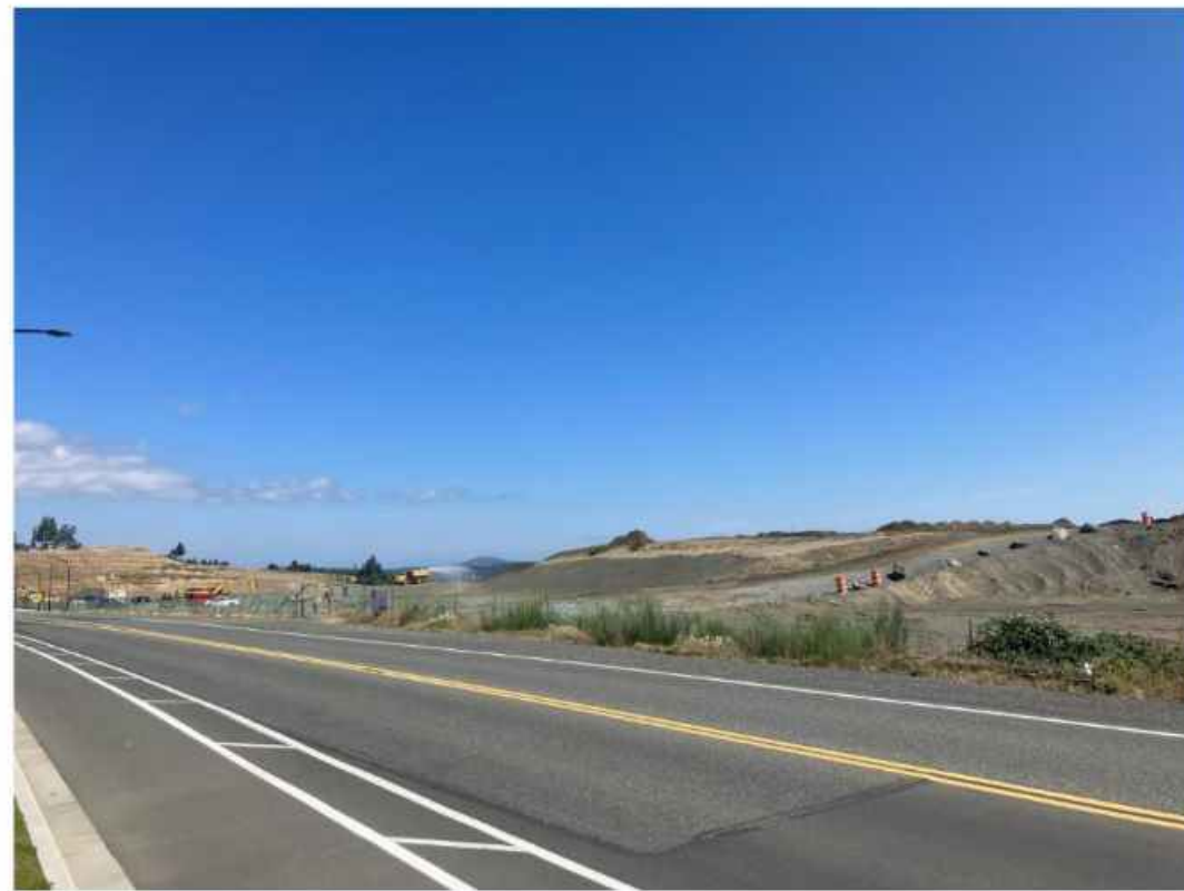
03 - VIEW FROM SOUTH-WEST - METCHOSIN ROAD
