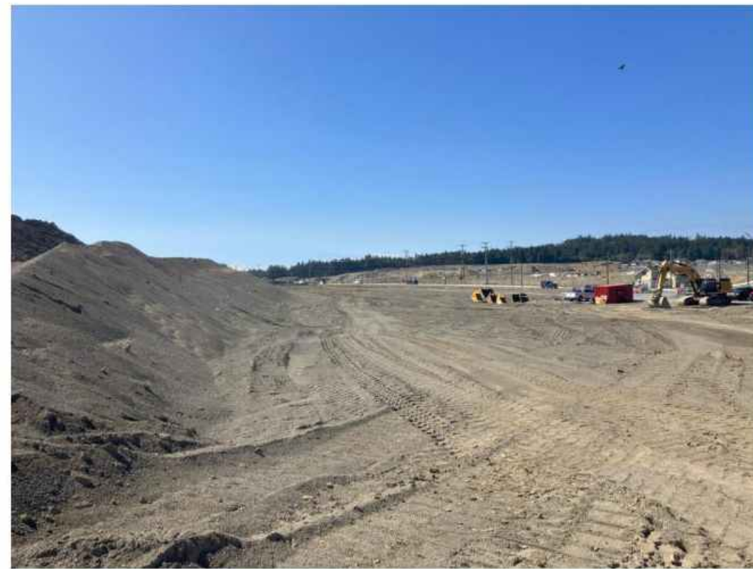
04 - VIEW FROM NORTH-EAST - SEABLUFF CRESCENT
