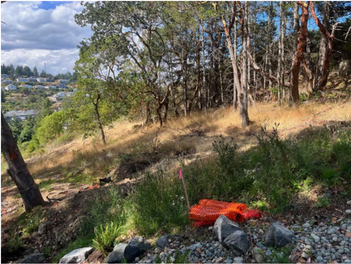
Photo 22. Looking west across the lower southwest steep slope of the property and desiccated plants.
