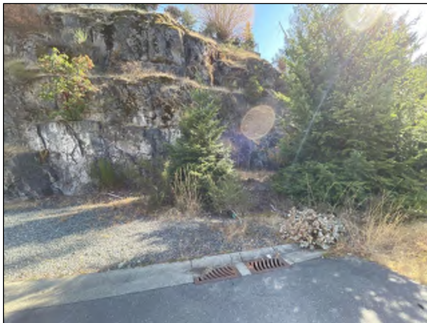
Site Photo 2: Showing Spotswood Terrace Road Dedication Rock Cutslope – Looking East
