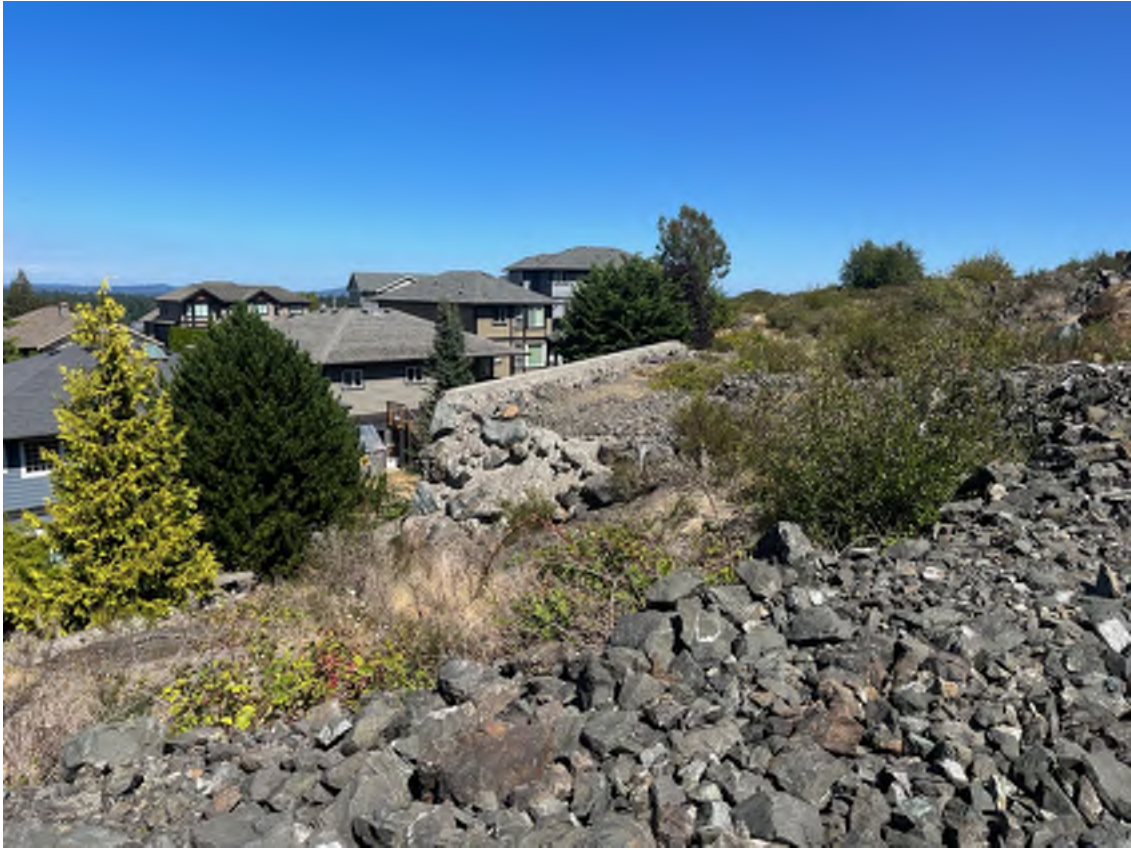
Photo 11. Looking at the Cottyn Way homes backing onto the property; stockpiles of blast rock dominate this portion of the property.
