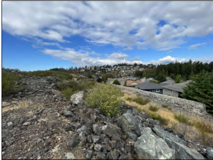
Site Photo 3: Showing Existing Fill At North End of Property – Looking Northwest
