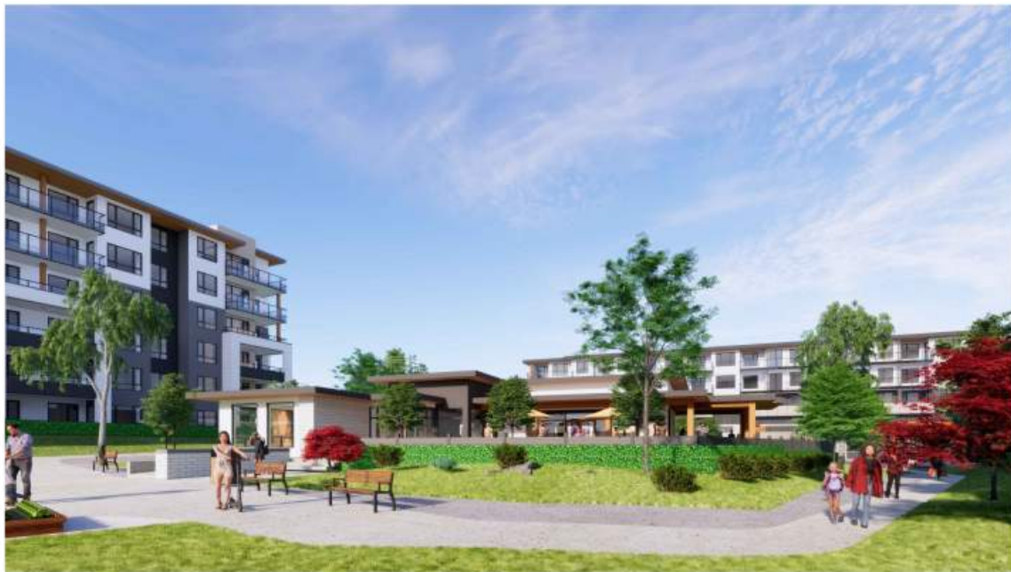
VIEW NORTH OF AMENITY BUILDING FROM INTERIOR COURTYARD
