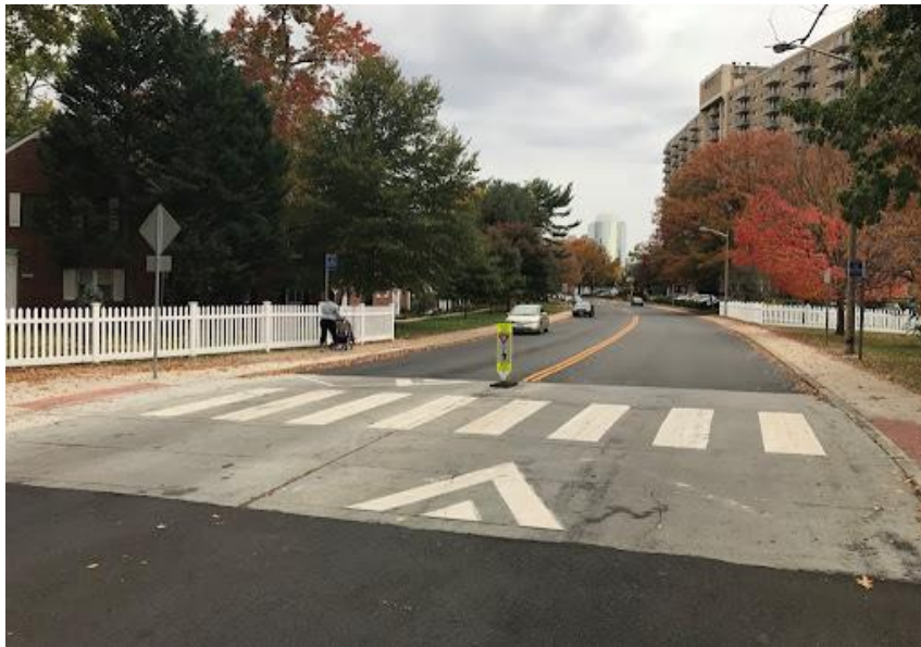
Figure 10: Example of Raised Crosswalk
