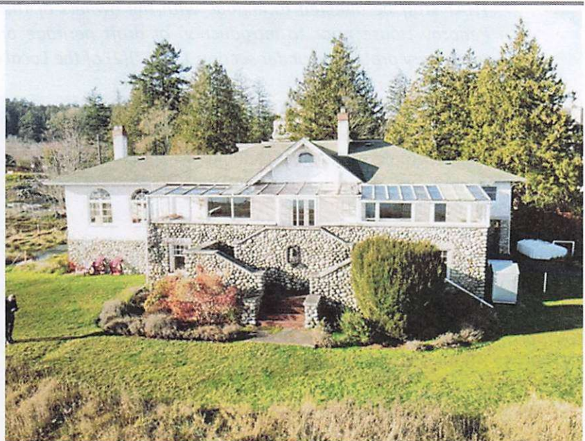
Figure 1 -View of the east façade of the Pendray House (source: CBRE)
