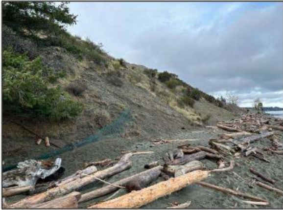
Figure 10 - View of bluff base at location P3
