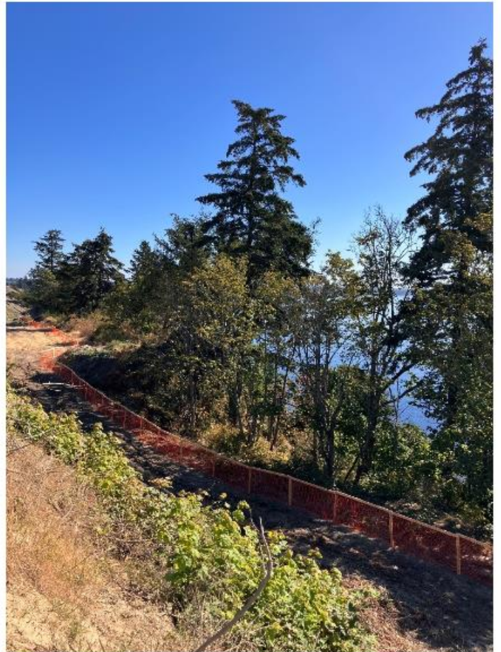
Figure 4 – Wood frame tree protection fencing at the edge of the eastern bluff
