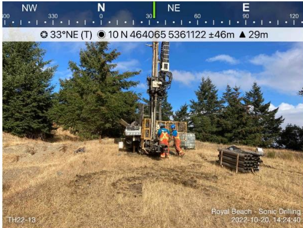
Photo 3. Drillwell advancing sonic drill at TH22-13.
