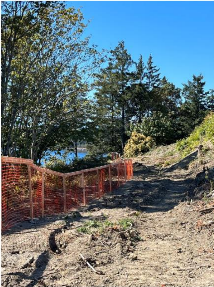
Figure 3 – Wood frame tree protection fencing at the edge of the eastern bluff
