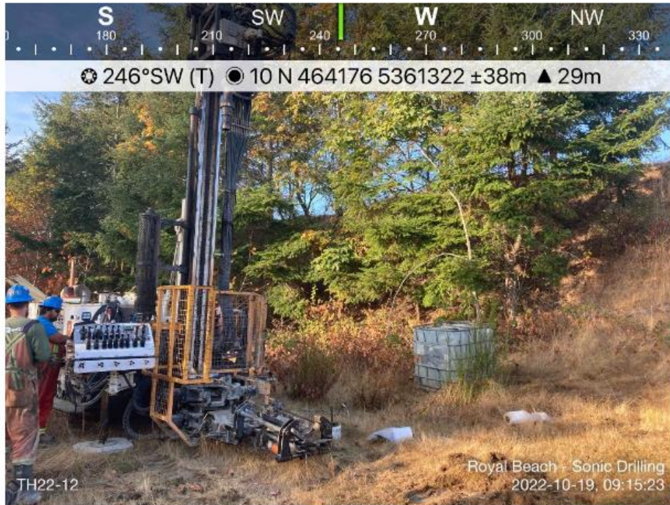
Photo 1. Drillwell advancing sonic drill at TH22-12.
