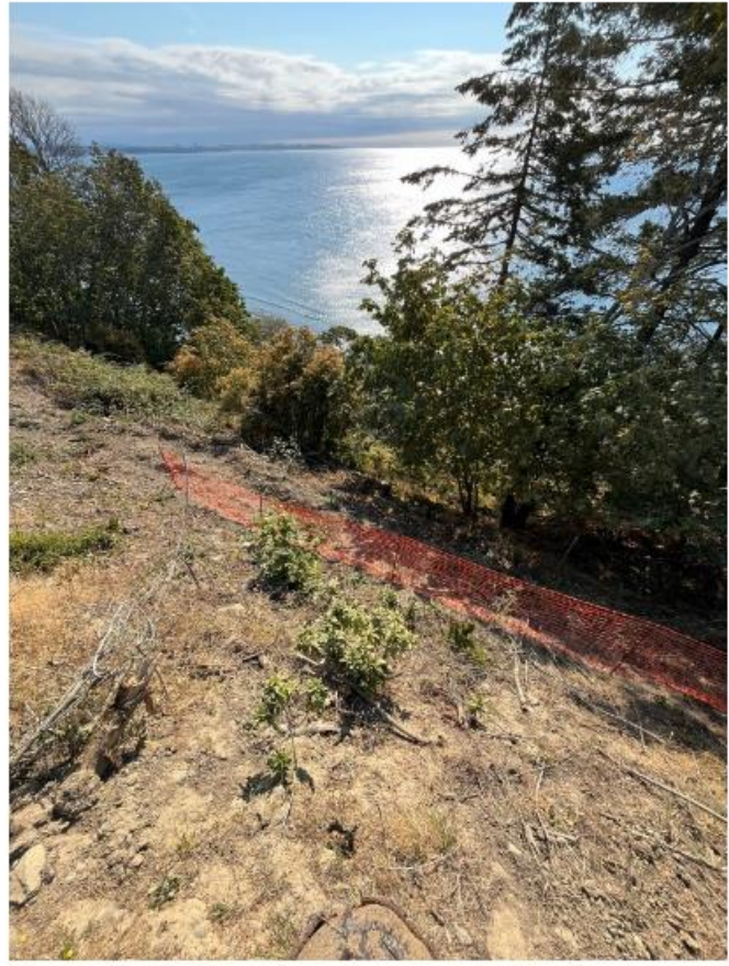
Figure 6 – T-post and mesh tree protection fencing on steep slopes above the eastern bluff
