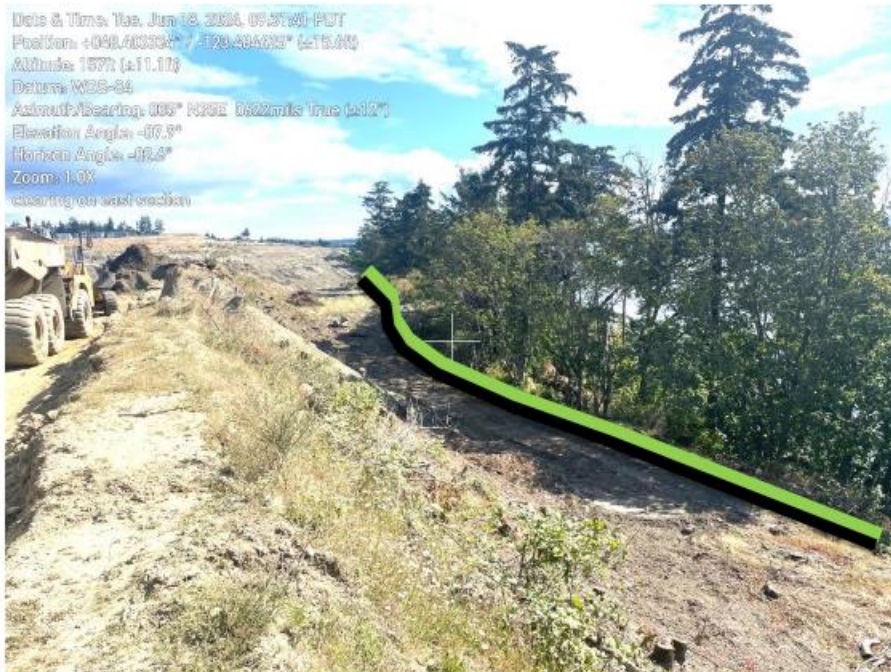
Photo 4. Silt fence (black) is to be installed inside the base of the tree protection fencing (green) as an additional protective measure against the migration of turbid stormwater offsite to the marine foreshore. Silt fencing installation can wait until mid-September.
