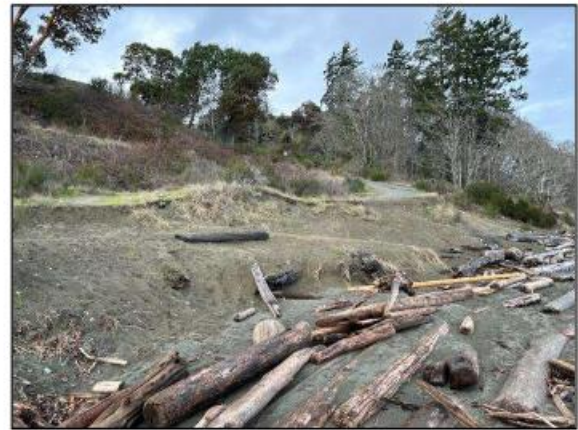
Figure 11 - View of bluff base at location P7
