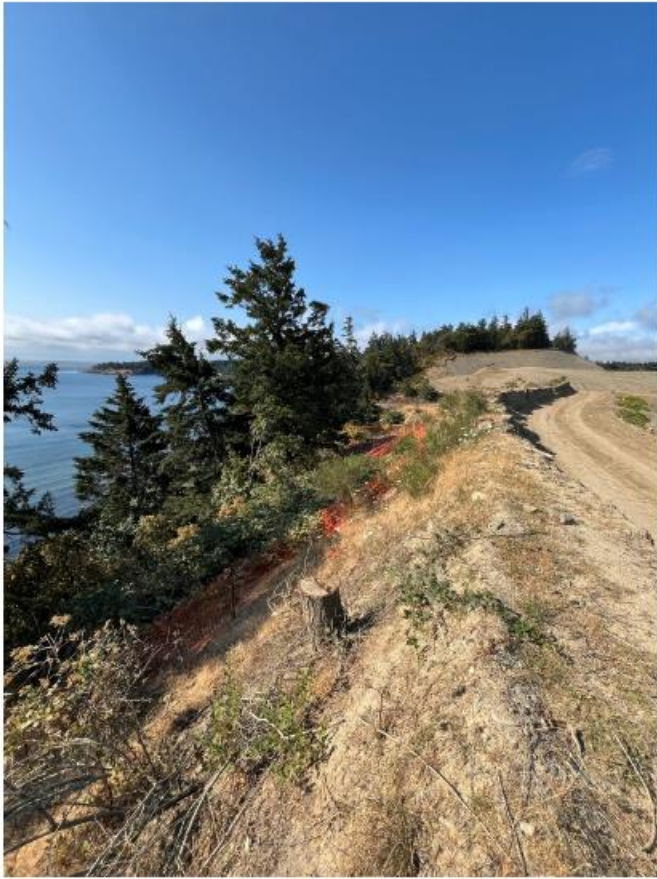
Figure 5 – Stumps remaining to be removed with arborist supervision
