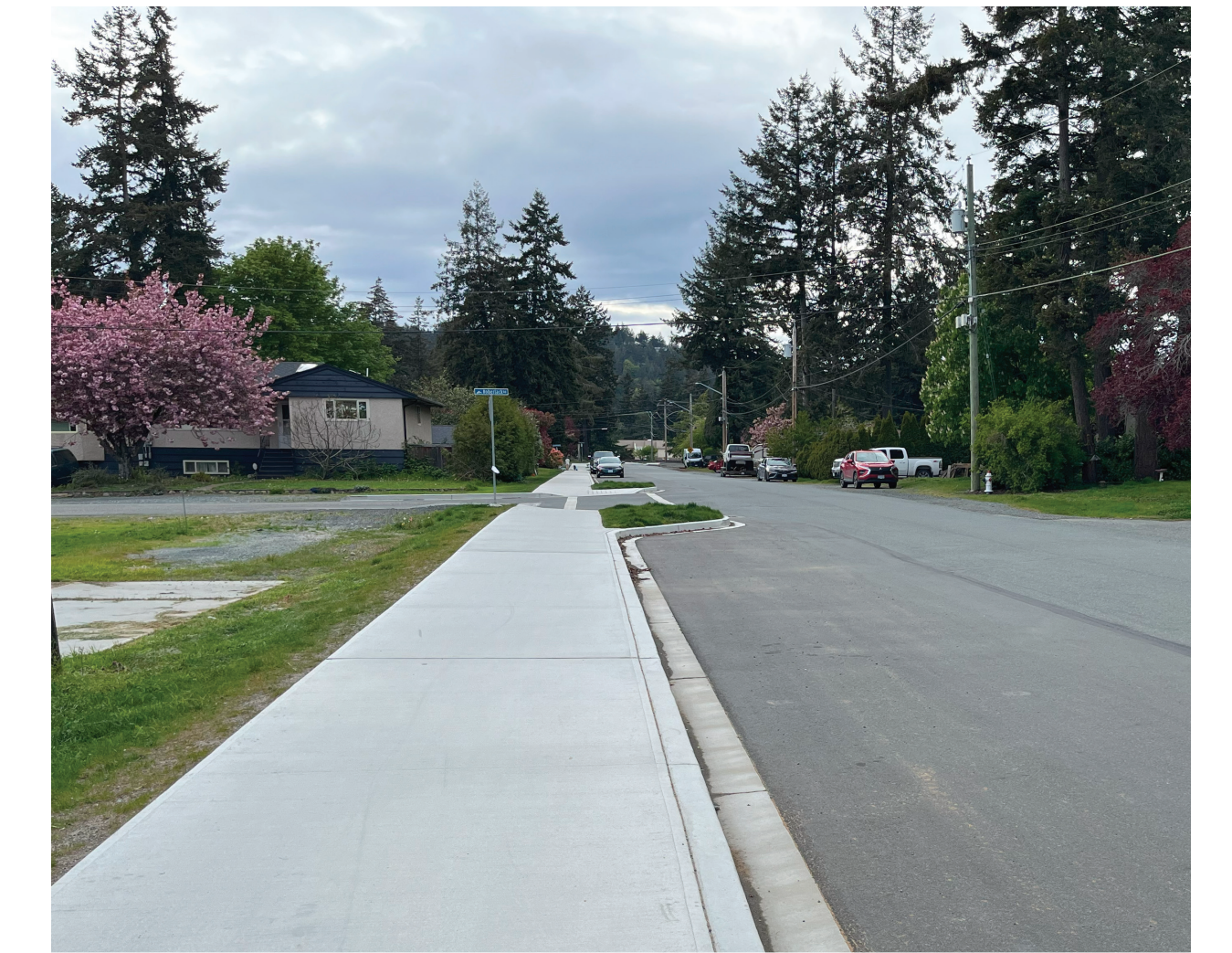
New sidewalks on Owens Road provide a safe walking connection to Colwood Elementary School and Dunsmuir Middle School
